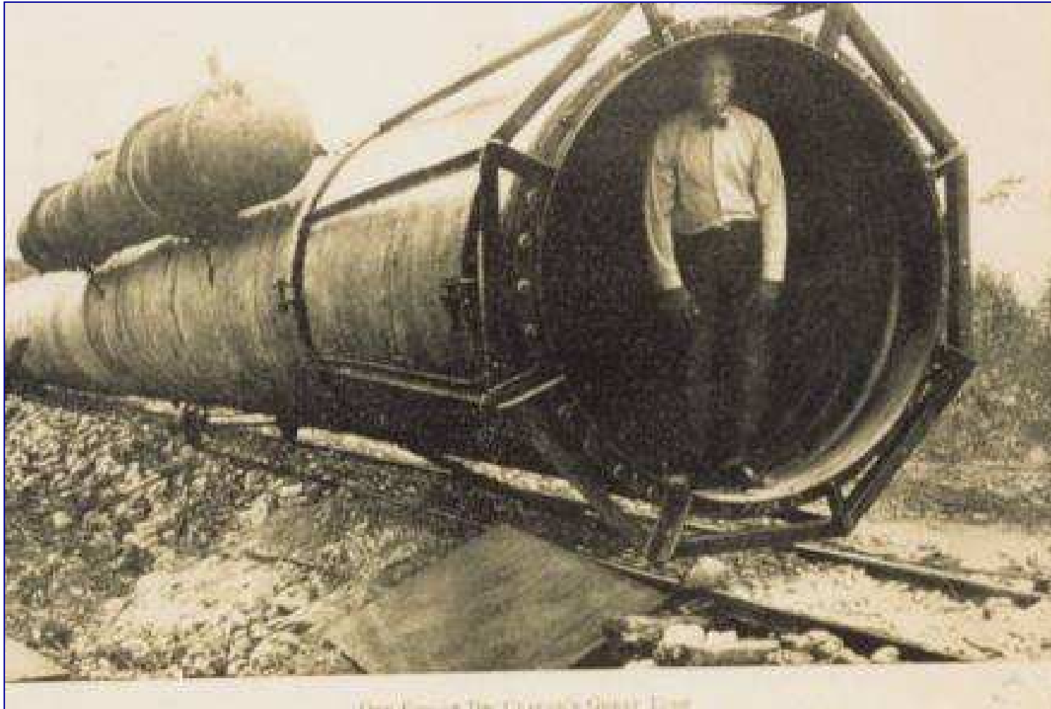
Corrugated Steel Cold Water Pipe Used by Claude in Cuba, 1930
